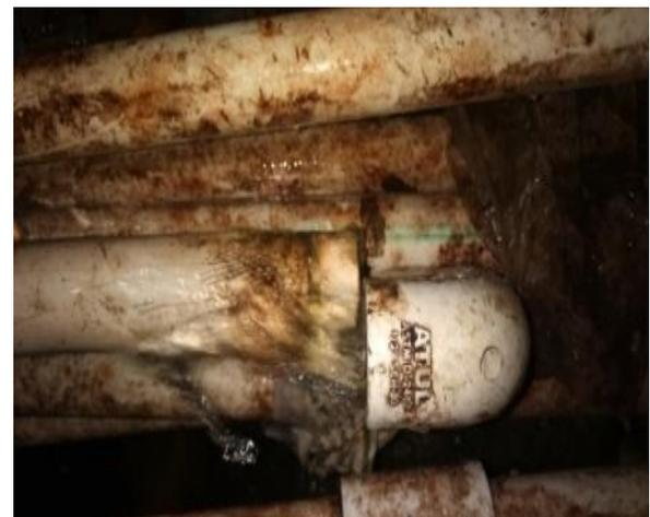
*Figure 40: Pipe Leakage Tajganj DMA*
