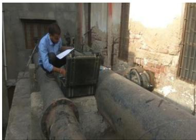
Five pumps are installed here, of which one was discarded and one was under maintenance at the time of audit. ESR filling and direct distribution are performed through dedicated sets of pumps and pipe lines.
