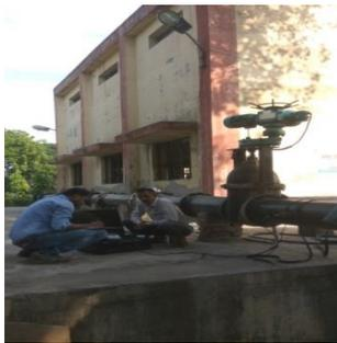
Total 3 pumps installed here (2W+1s) pump running time is not fixed but run 6 hour per day
