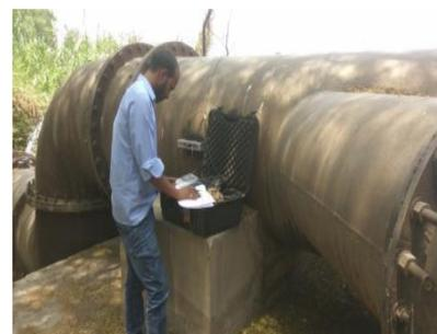
As seen in flow mesurment activity(Pump No-2), the average flow to Jeoni Mandi WTP from Raw water New intake well 2095.5 m<sup>3</sup>/hr and hence Inlet Supply to WTP is 42.36MLD.
