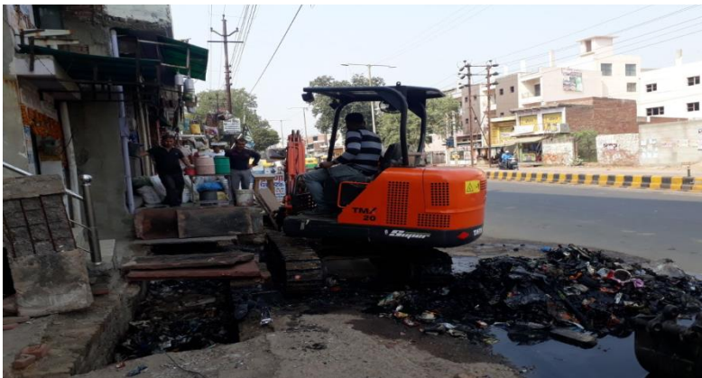
Drain Cleaning by Machine
