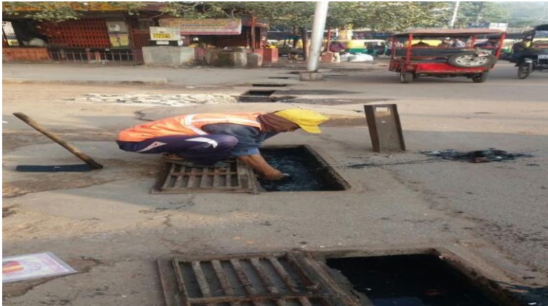
Drain Cleaning by Manually
